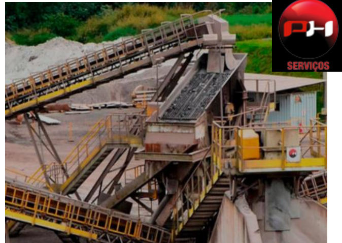
PH Slag Processing Plant
