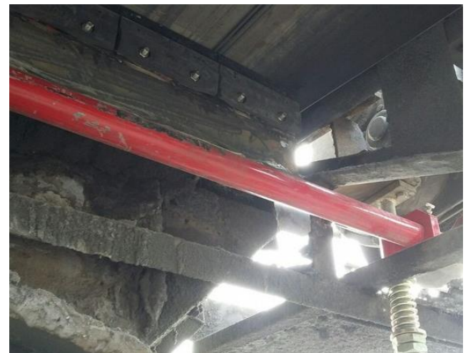
Condor PD Secondary modified at site
