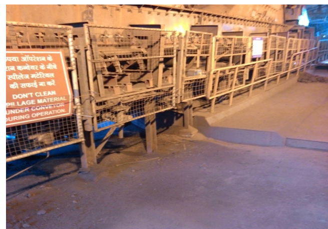
Transfer Point area after a week from the date of installation
