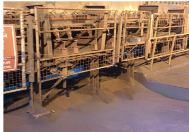
Transfer Point area on the date of installation, after cleaning
