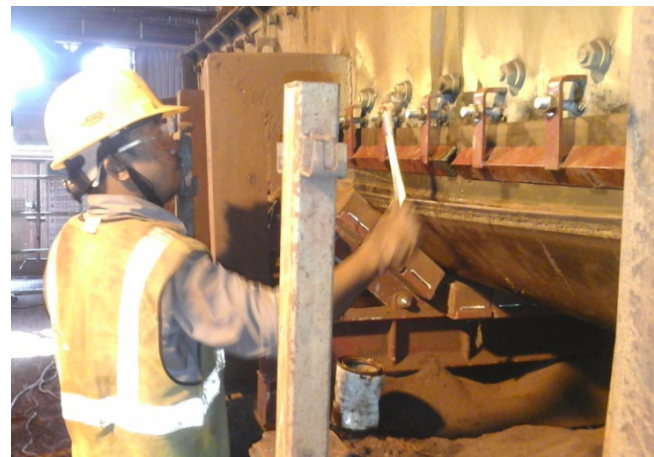
Thejo's technician installing TWINLIP seal
