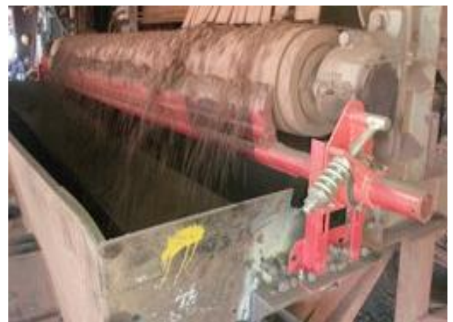
Installation at JSW Ispat, Mumbai-4000mm B/W
