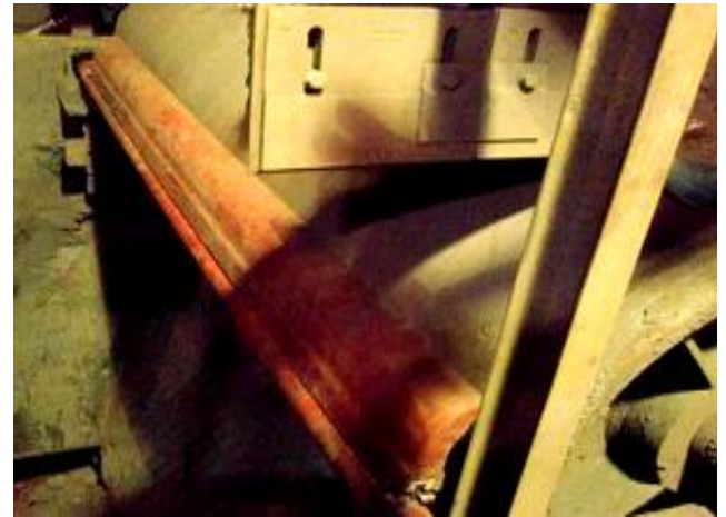
CONDOR 4400mm Primary Installed on the discharge pulley
